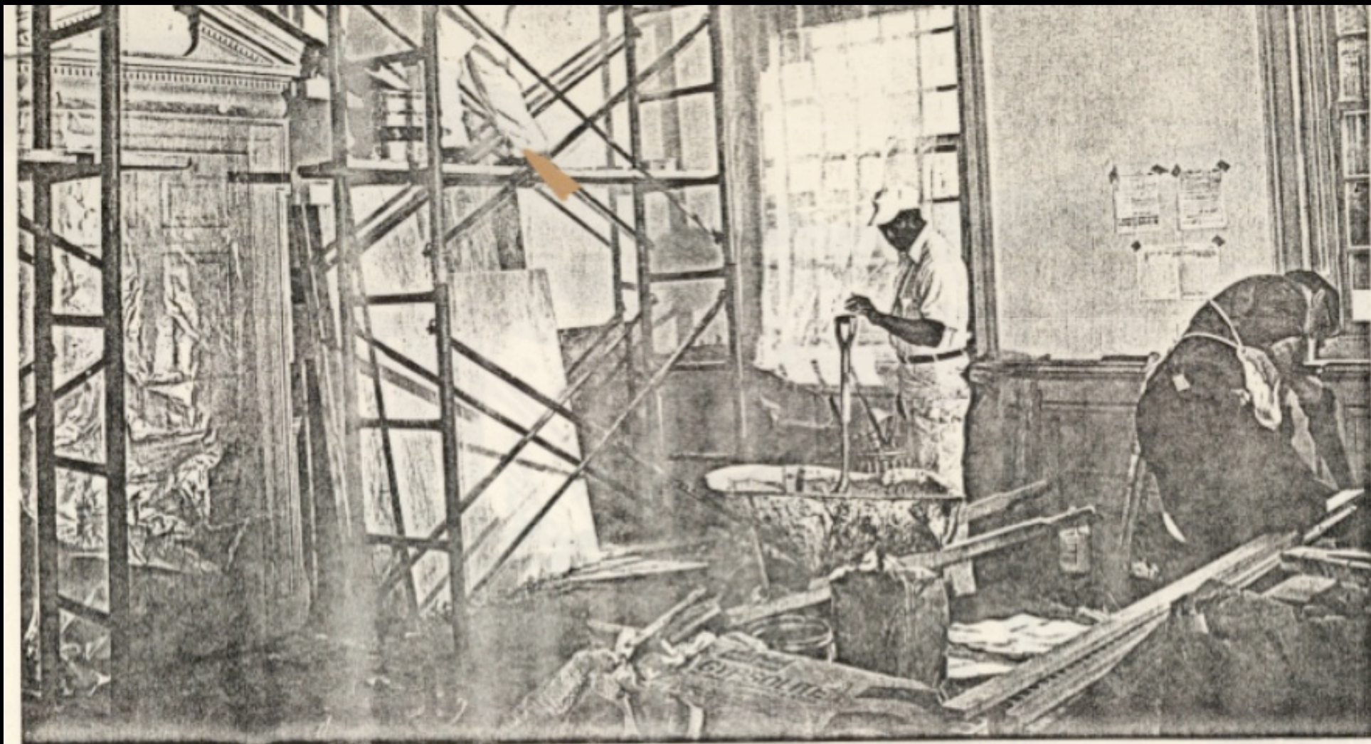
(9) A plasterer applies a rough coat to the ceiling of the reception room, while a carpenter (right) removes the sag in the dentils prior to replacing them on the north wall of the reception room.
