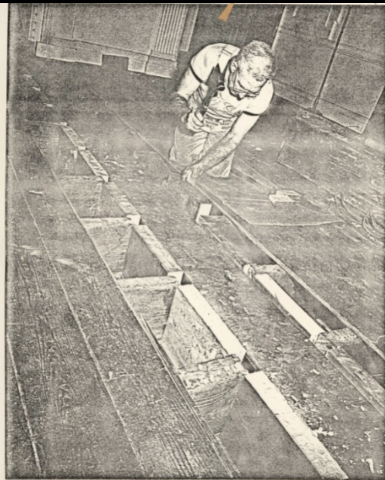
(7) A carpenter fits spacers between the joists. Both spacers and joists rest on an oversized steel plate welded to the bottom of the I-beam. Later angle irons, fastened with bolts and lag screws, bonded joists and spacers. (Photo 3/6/ 78)
